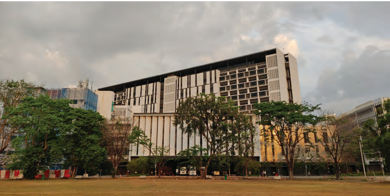
The hospital complex from the main road; the Clinical block is in the foreground with the Ward block in the background.
