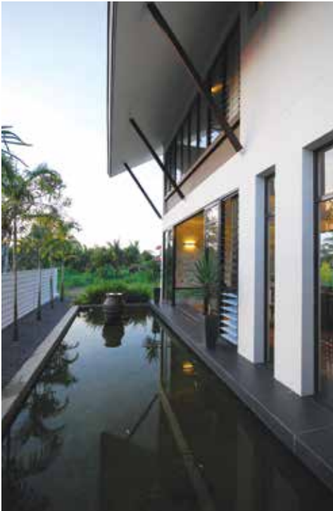
The roof eaves are extended lower on the west facing side of this house. (1-tree House by Design Network Architects.)
