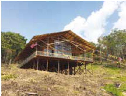
The church building was completed after 15 days.
