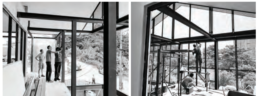
The extension was primarily built in steel to reduce the loading and increase permeability and ventilation.
