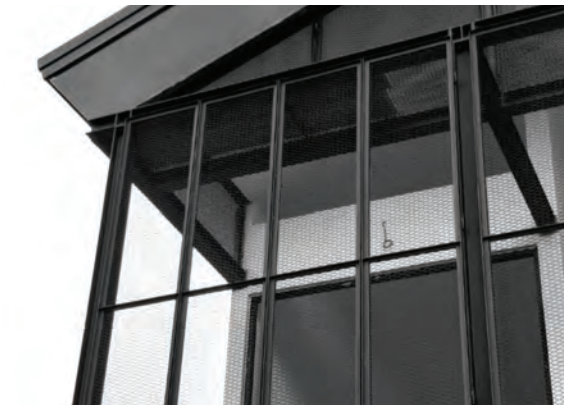
The extension was primarily built in steel to reduce the loading and increase permeability and ventilation.
