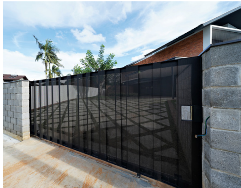
LEFT The front gate of folded perforated sheets allows visual connection to the house and air to pass through
