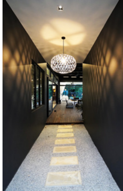
Walkway leading to the central terrace from the service area. This is one of the two links that constantly draw air into the space beyond, creating a wind tunnel effect
