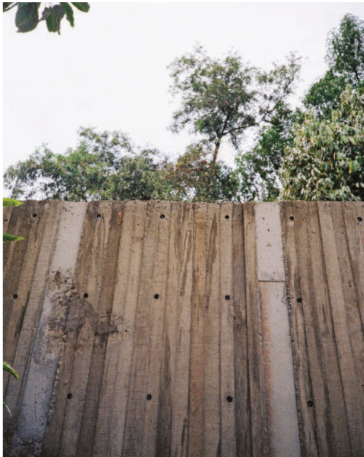
The off-form concrete of the TV room.
